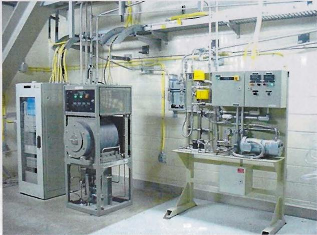
Fig. 9 The Stack Monitoring System at the Tritium Removal Facility
